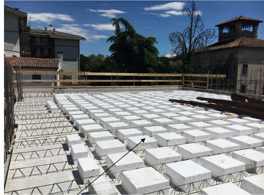
Solaio Dual Solution
